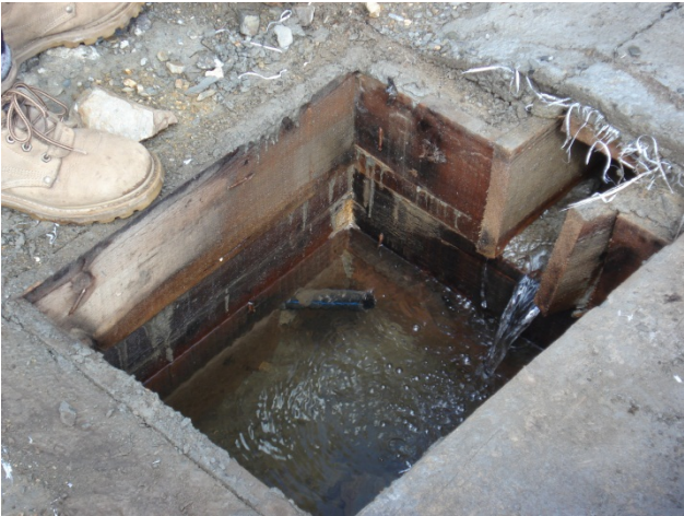
Figure 2: Lower spring source ( S_1 ) has a discharge of 17 liters per minute.
