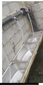
Challenge: The school reported leaky water taps in spring 2014 and we believed it was due to the freezing of water in the outdoor taps. Ouyang and Tim replaced the water taps and repaired the pipe insulation when they visited the school in September 2015 – THANK YOU guys!
